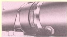
The design, fabrication and erection of Penstock Specials with extra high tensile steel to withstand very high pressure is a challenging job. IHP technicians have, during past several years successfully designed, fabricated and erected various
